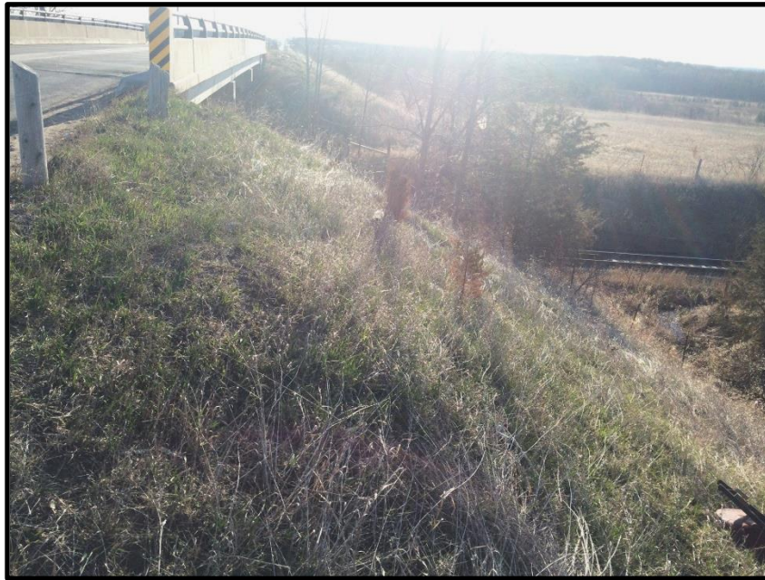
Photograph 2: Looking East on South Side
