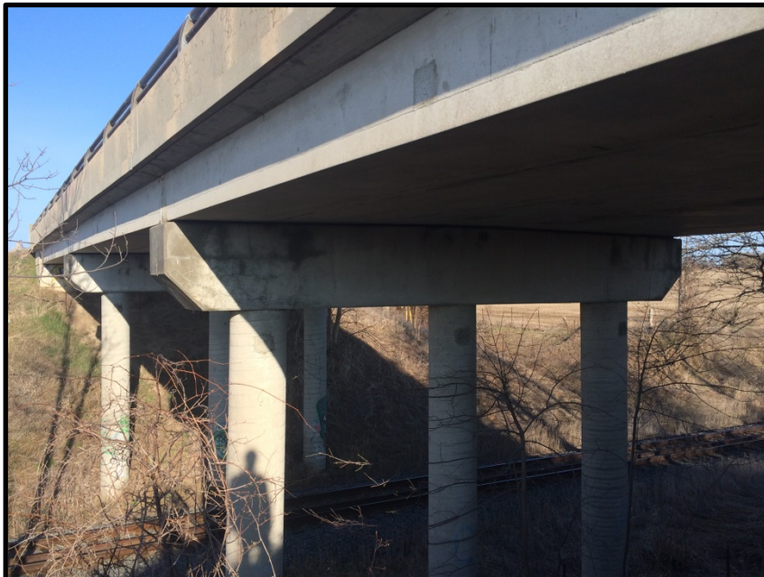
Photograph 1: Looking West from South Side
