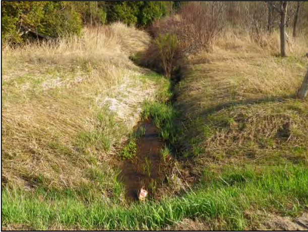
Crossing E: Looking south (downstream) from 6 th Line at a Tributary of Innisfil Creek.
