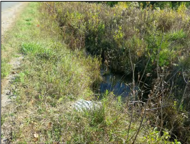
Looking east along the south side of 6 th Line, approximately 1.2 kilometers west of St. Johns Road.
