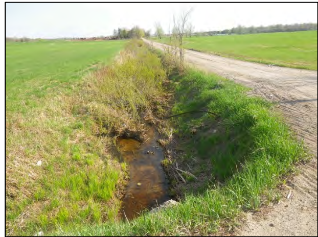
Crossing F: Looking south (downstream) from 6 th Line at a Tributary of Innisfil Creek.
