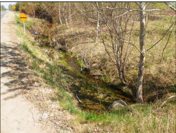
Looking southeast from 6 th Line, along where Cedar Creek exits the study area.
