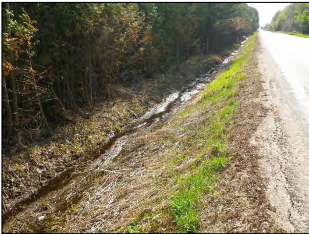
Crossing H: Looking west from south (downstream) of 6 th Line at a Tributary of Banks Creek.
