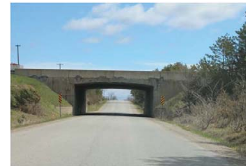
6th Line Bridge as viewed from west
