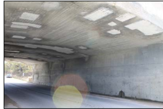
Underside of 6 th Line Bridge
