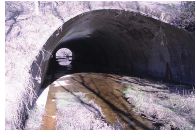
Highway 400 Concrete Arch culvert C-55 – upstream face. The Creek flows cross the concrete invert slab as a thin film
