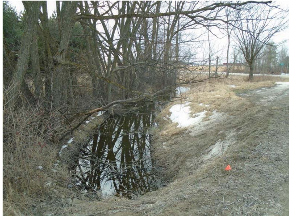
Photo 3: Innisfil Creek crossing 6th Line (north)
