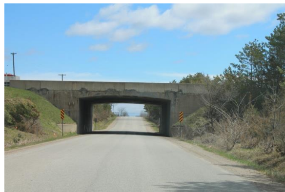
Photo 3: View of the bridge looking west
