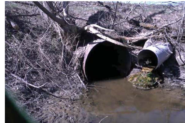
1.7 m diameter culvert conveying Innisfil Creek (left). Smaller CSP conveys flow from north ditch (across) – note deposits at outlet
