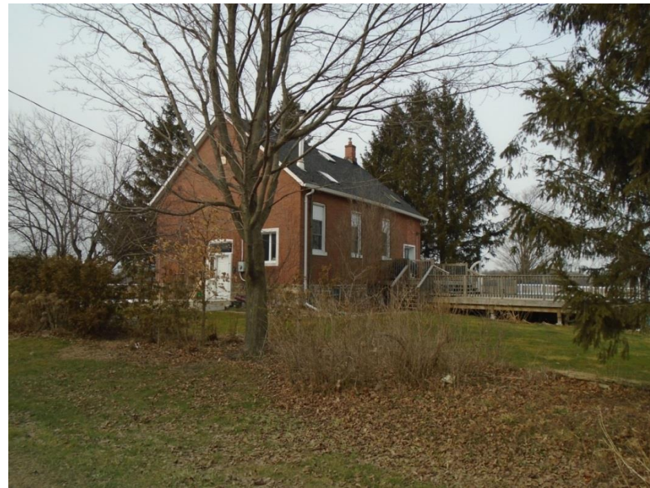
Photo 5: Former Schoolhouse (3654 6th Line)
