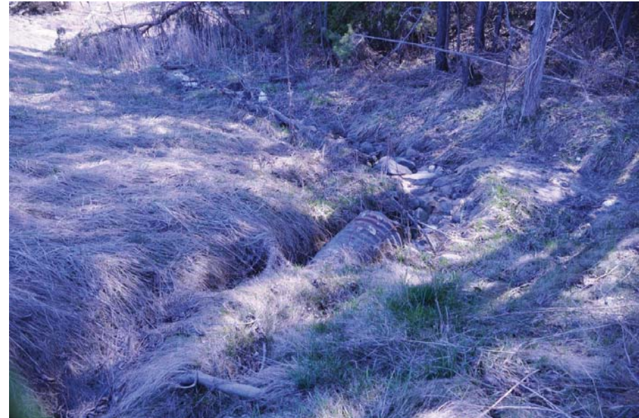
Photo 2: Corrugated steel pipe culvert
