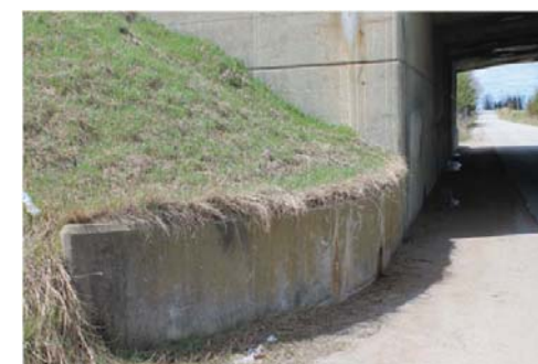
Detail of 6th Line Bridge
