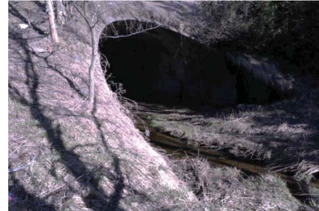
Highway 400 Concrete Arch culvert C-55 – upstream face. The Creek flows cross the concrete invert slab as a thin film
