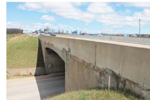
6th Line Bridge as viewed from side of Highway 400
