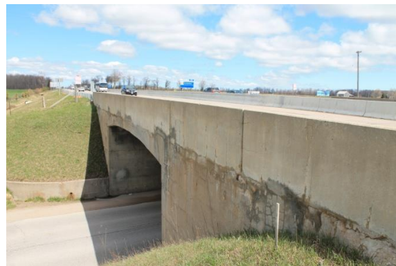
Photo 2: View of the bridge from Highway 400
