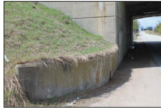
Detail of 6 th Line Bridge abutment
