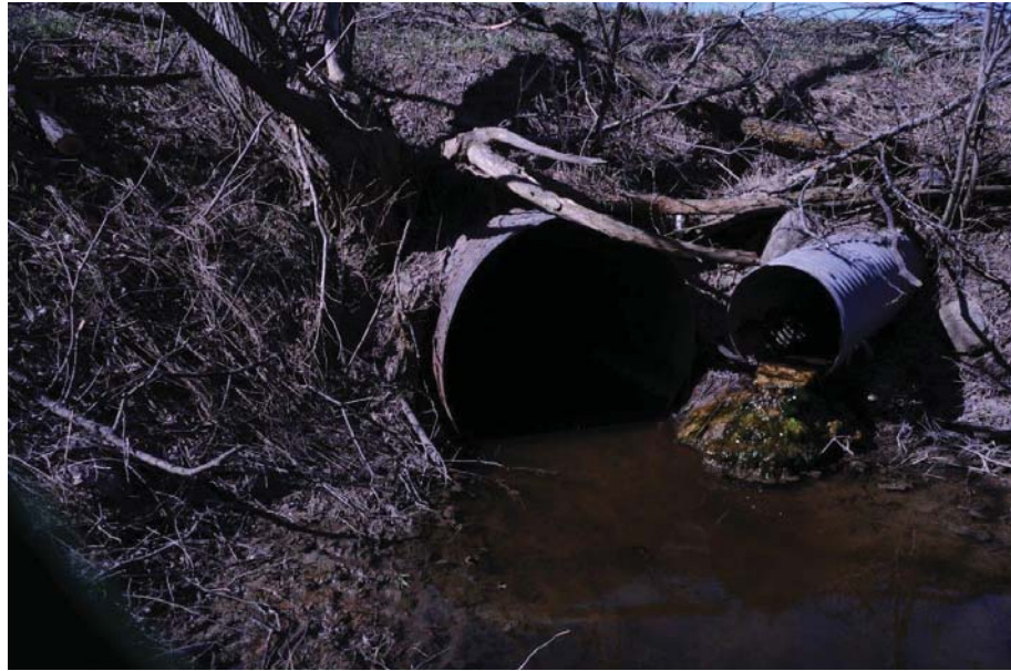
Photo 10: Deposit, south of 6 th Line, west of Highway 400
