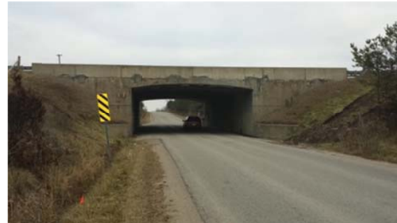
Photo 2: Current Overpass Structure
