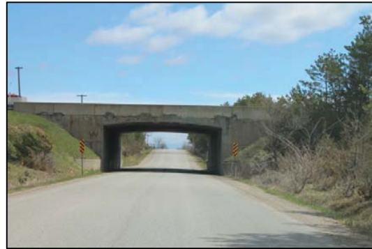
6 th Line Bridge as viewed from the west
