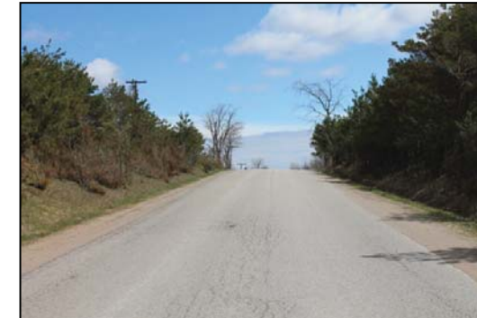
6 th Line looking west from the bridge structure
