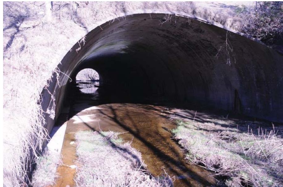
Photo 3: Concrete culvert, view eastward
