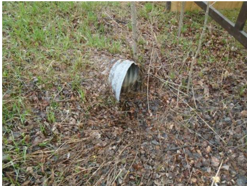
Photograph 8: Existing CSP 550 metres east of Webster Boulevard
