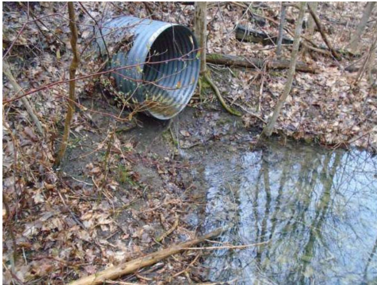
Photograph 4: Existing CSP 470 metres east of 20 th Sideroad
