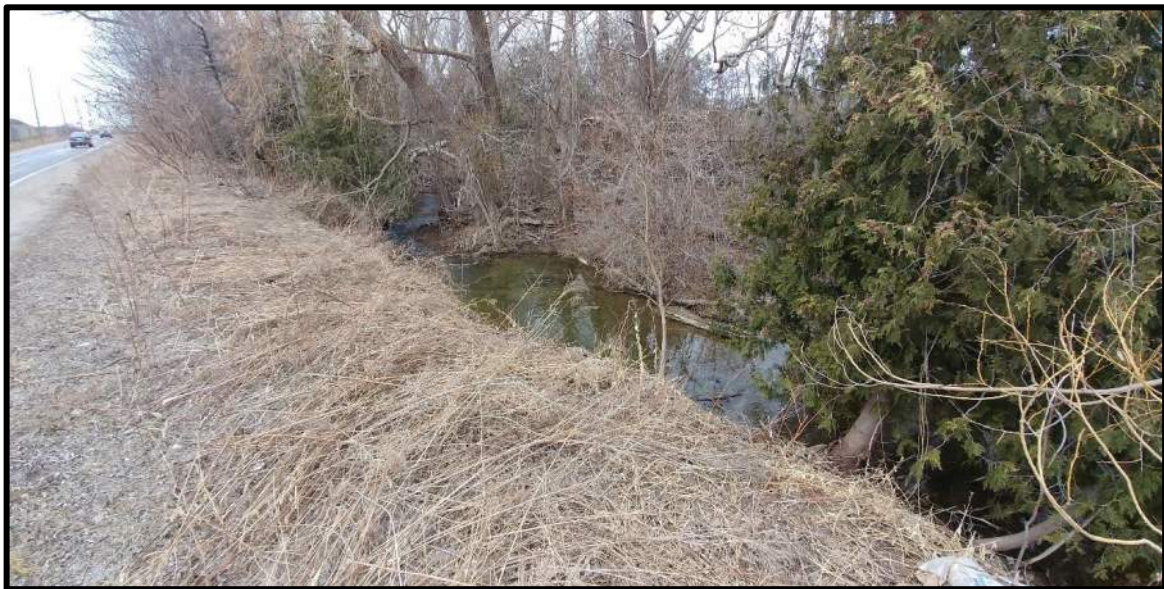
Photograph 1: Point of initial impingement
