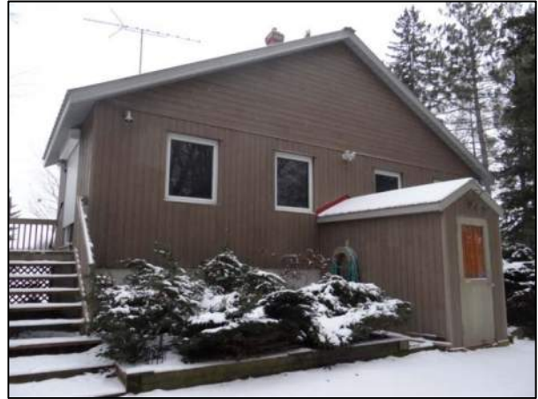
Plate 10: East elevation, looking northwest.
