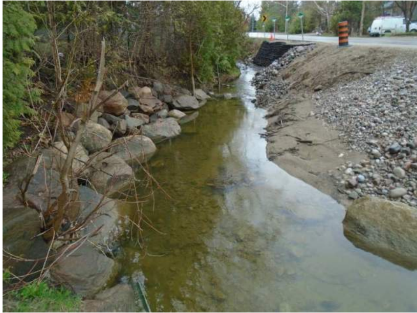
Photograph 13: Outfall at St. John's Road/7 th Line culvert crossing
