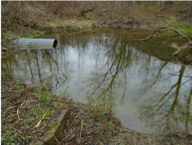
Photograph 3: Existing corrugated steel pipe (CSP) 300 metres east of 20 th Sideroad
