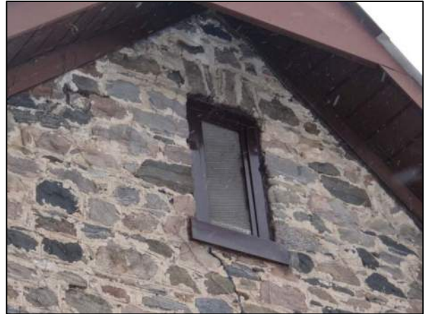
Plate 4: West gable end window.
