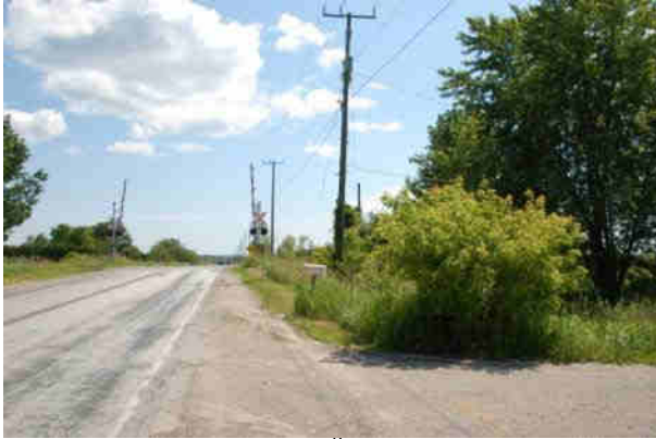
Plate 7: Northeast view of 7 th Line; Areas on both sides of disturbed ROW up to the railway corridor exhibit potential, require Stage 2 test pit survey to the north and south, and pedestrian survey to the south
