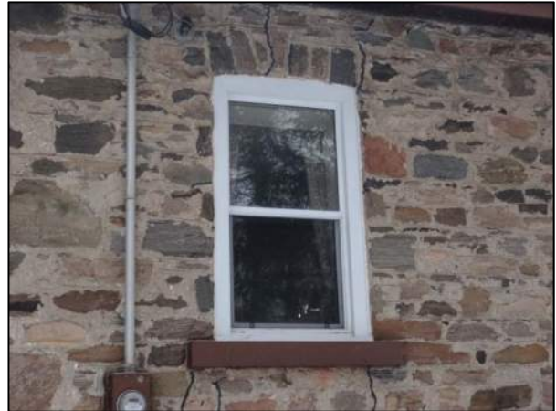
Plate 12: Window on north elevation, looking south.
