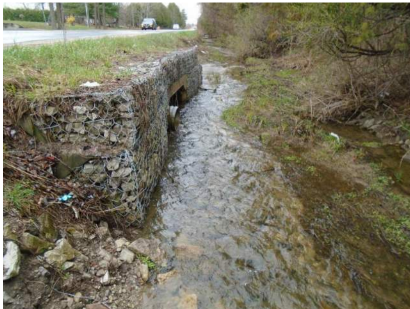
Photograph 10: Existing CSP at Quarry Drive crossing 7 th Line
