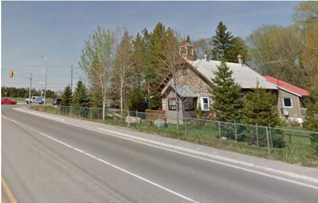
Figure 15: Former School at 1494 7 th Line Looking North In Relation to Intersection at 7 th Line & 20 th Sideroad
