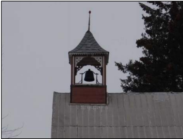
Plate 13: Belfry at west end of structure, looking north.
