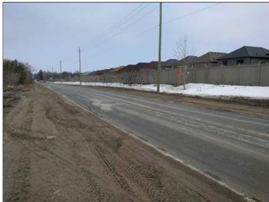
Existing 7 th Line Corridor with Gravel Shoulders and No Sidewalks
