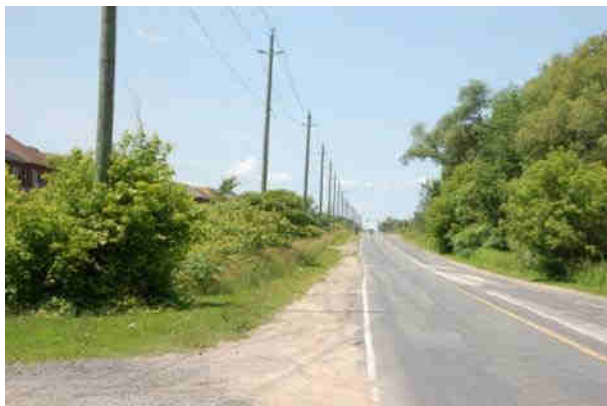
Plate 17: Southwest view of 7 th Line; Area on both sides of disturbed ROW exhibits potential, requires Stage 2 test pit survey
