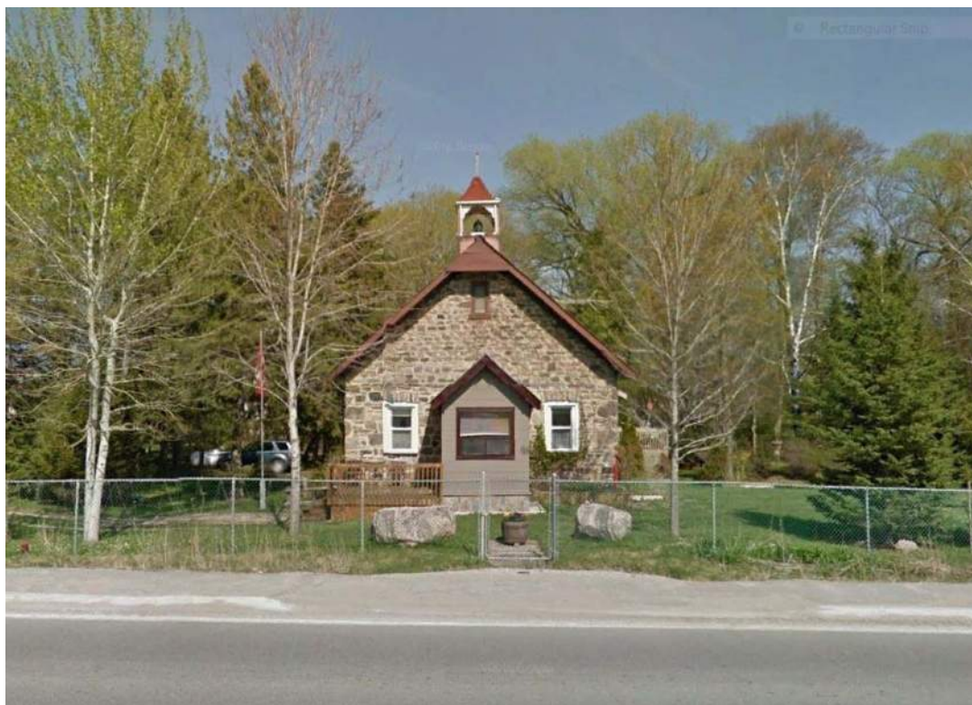
Figure 8: 1497 7 th Line – Former Nantyr School (now residence)
