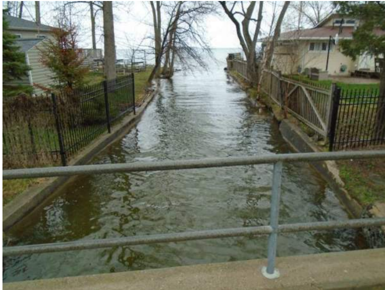
Photograph 14: Banks Creek outflow into Lake Simcoe
