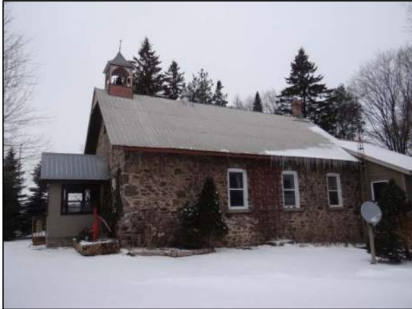
Plate 6: South elevation, looking north.
