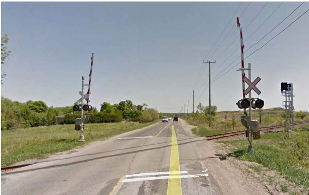
CN Rail Crossing Looking East
