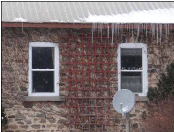
Plate 8: Windows on south elevation, looking north.
