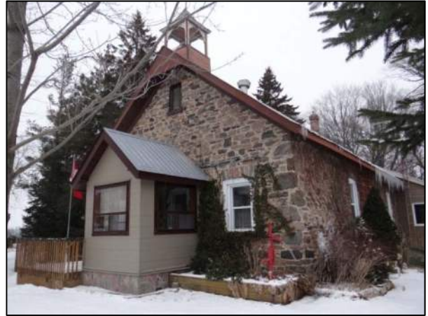
Plate 2: West elevation, looking northeast.
