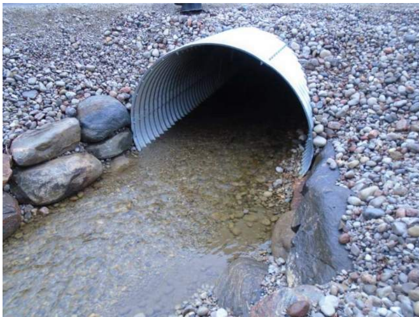
Photograph 12: Existing culvert at St. John's Road crossing 7 th Line
