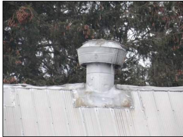
Plate 14: Woodstove chimney, looking north.
