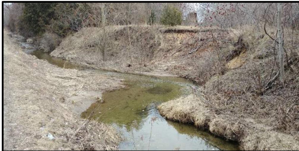
Photograph 3: Bank erosion at apex of channel pinchpoint
