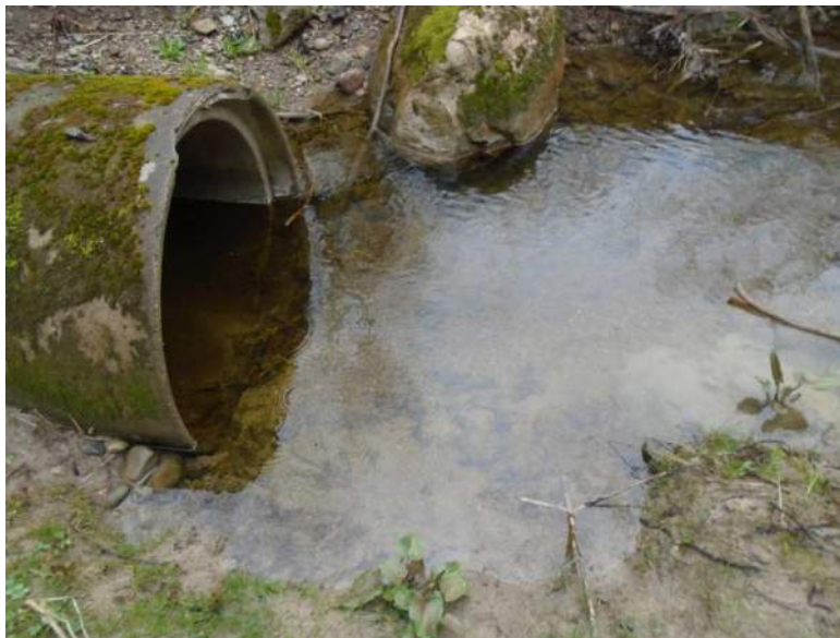
Photograph 2: Existing culvert 200 metres east of 20 th Sideroad
