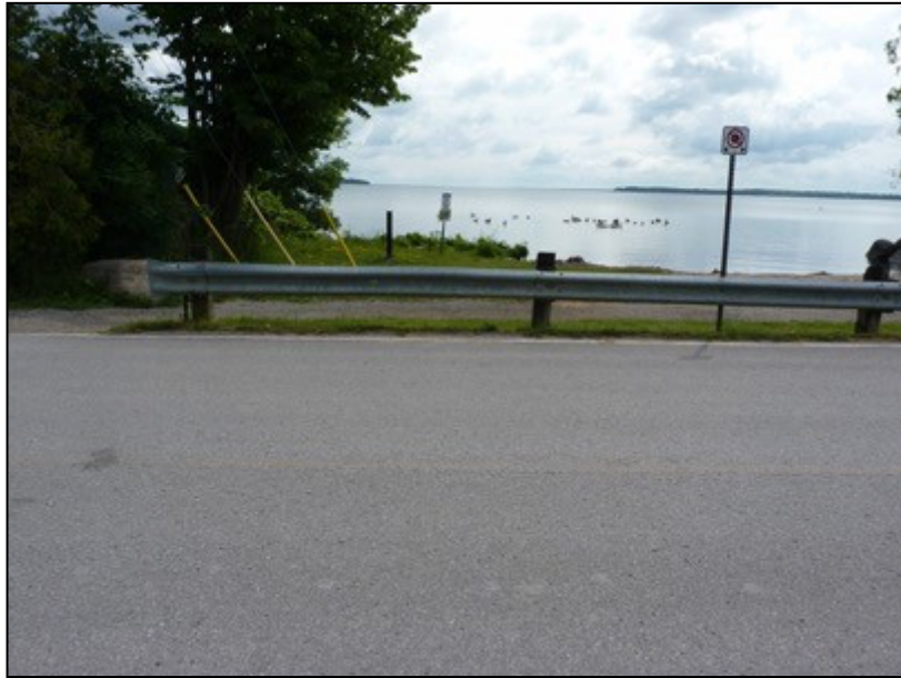
Image 1: Shows disturbed areas at Roberts Road Outlet.
