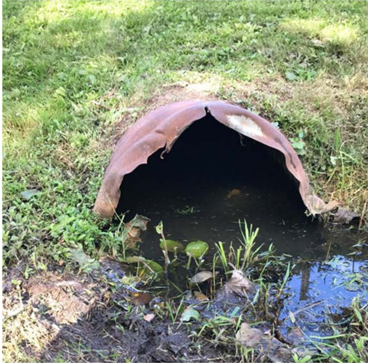
Photograph 17: Outlet of 600 mm Dia. Buchanan Street/Crystal Beach Road Culvert
