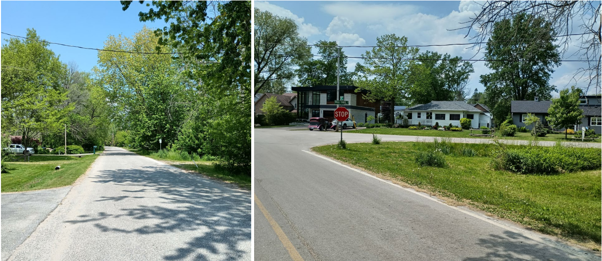
Figures 5 & 6: Existing verge and ditch along the west side of Tall Tree Lane and intersection of Tall Tree Lane and Crystal Beach Road.
