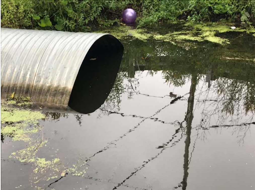
Photograph 13: Goodfellow Avenue 2100 mm Dia. Culvert Crossing Outlet
