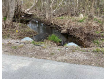
Buchanan St Culvert Crossing, Looking Downstream
