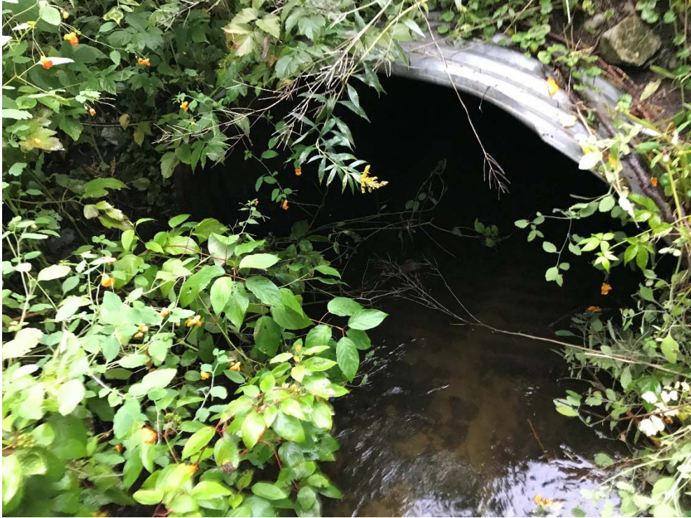
Photograph 9: Tall Tree Lane 1800 mm Dia. Culvert Crossing Inlet
