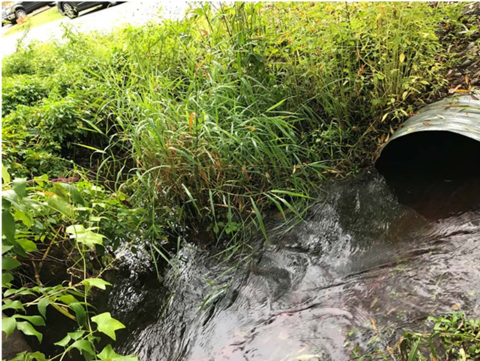
Photograph 4: Buchanan Street Twin 900mm Dia. Culvert Crossing Outlet
