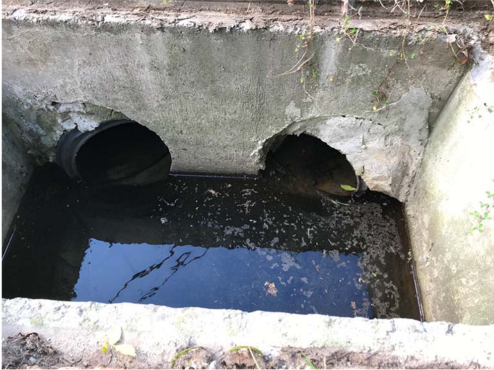
Photograph 7: Tall Tree Lane (Outlet #2) Ditch Inlet Catch Basin Structure inlets
