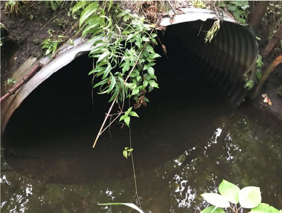
Photograph 10: Tall Tree Lane 1800 mm Dia. Culvert Crossing Outlet
