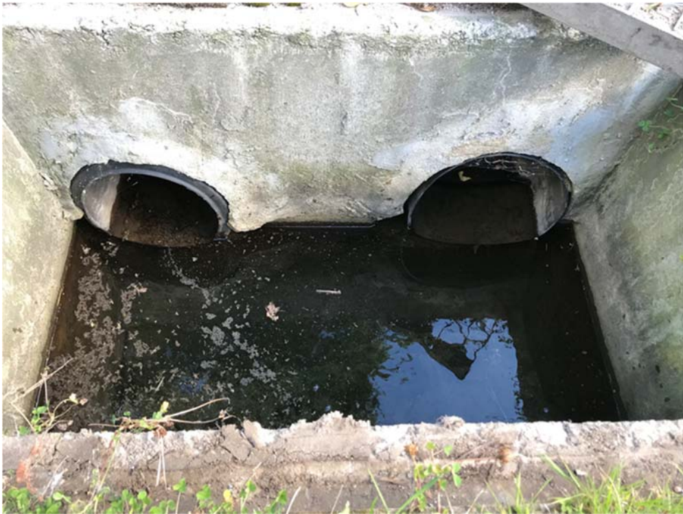
Photograph 8: Tall Tree Lane (Outlet #2) Ditch Inlet Catch Basin Structure inlets
