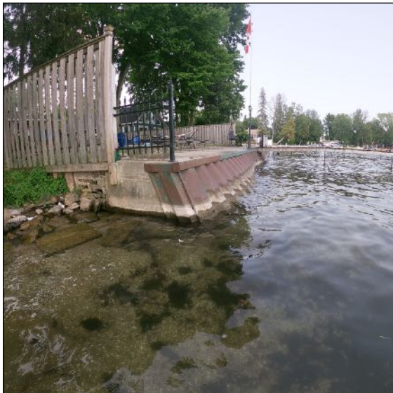
Image 3 : Steel piling and associated cribwork adjacent to the marine study area.
