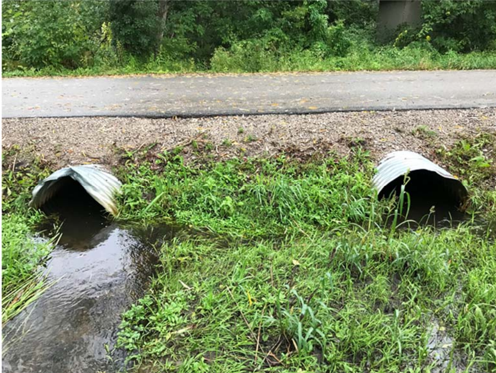
Photograph 3: Buchanan Street Twin 900mm Dia. Culvert Crossing Inlet
