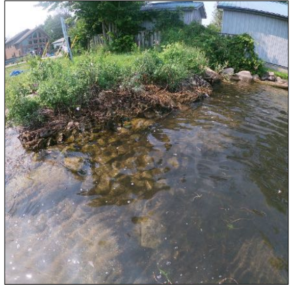
Image 2: Existing impacts and gabion wall.
