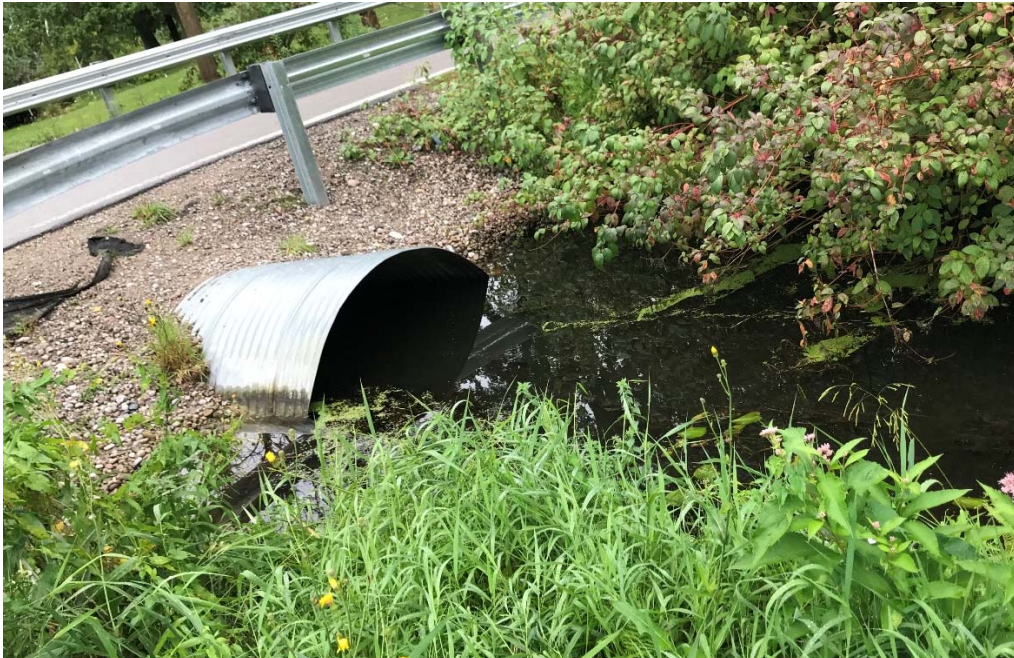
Photograph 12: Goodfellow Avenue 2100 mm Dia. Culvert Crossing Inlet
