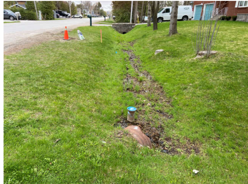
Existing Hartley Rd Culvert Outlet (Looking South on Crystal Beach Rd)
