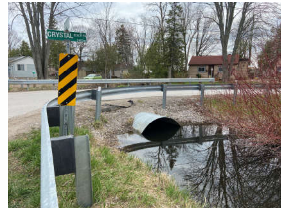
Existing Crystal Beach Rd Culvert
