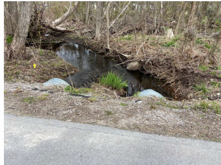
Buchanan St Culvert Crossing, Looking Downstream
