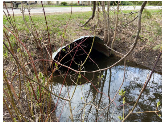
Existing Tall Tree Ln Culvert
