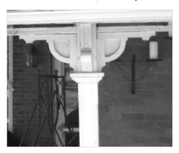
Apply traditional joining details. The use of dovetail, tenon and mortise, dowels, and splines is more preferred over metal fasteners during repair
