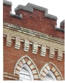
Dichromatic brickwork achieved by using red and buff bricks.
