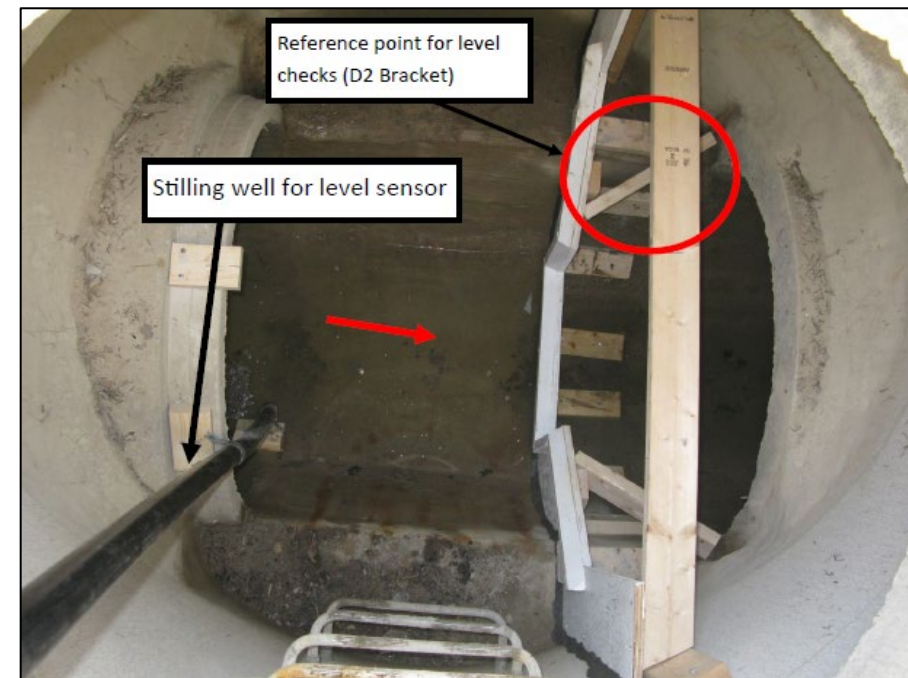
Photograph 21: SWMF #6 (South Inlet Weir)
