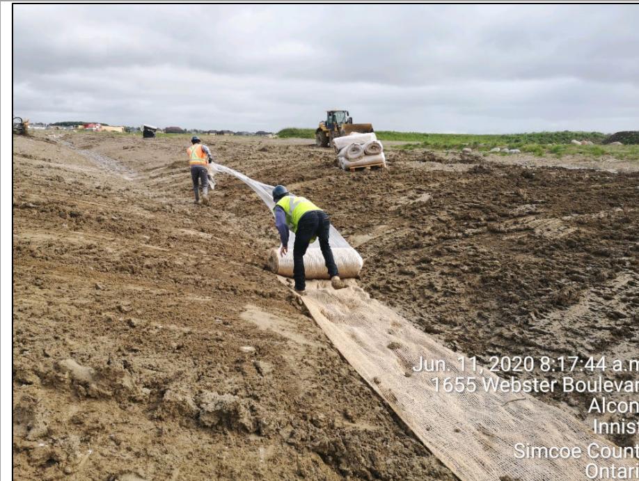
Photograph 7: Installation of Treated Jute at SWMF #7 (west channel)
