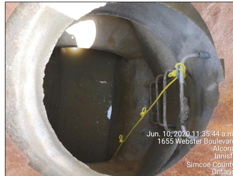
Photograph 5: Securing of Gel Flocculant Blocks (WLB 494 & WLB 360) at select MH ladder rung
