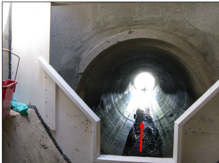
Photograph 20: SWMF #6 (South Inlet Weir)
