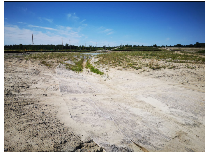
Photograph 15: Treated Jute fully saturated with Sediment
