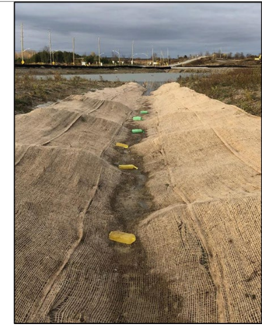
Photograph 11: Final Installation Configuration at SWMF 7 (Treated Jute, Gel Flocculant Blocks and Rock Check Dams)
