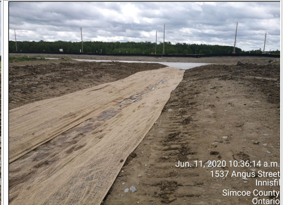
Photograph 8: Fully lined channel with Treated Jute at SWMF #7 (west channel)
