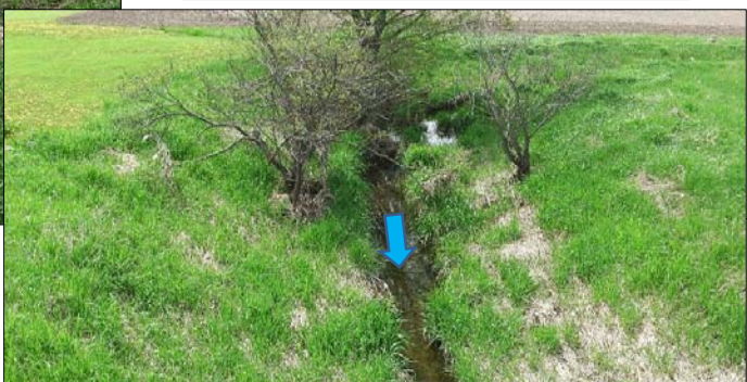
▼ Overview looking upstream from 10th Line
