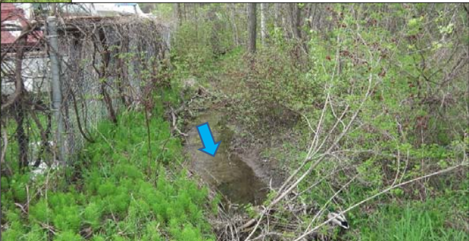
▼ Overview looking upstream from a point above 25th Sideroad
