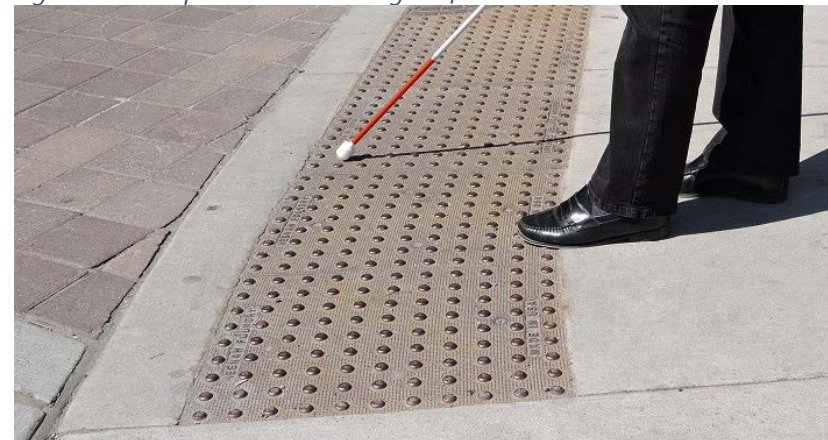
Figure 33: Sample Tactile Walking Surface Indicator
